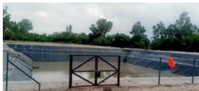
Construction of Surface Rainwater Storage Ponds in plant premises progress
