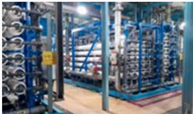
RO installed on treated effluent and other process streams
