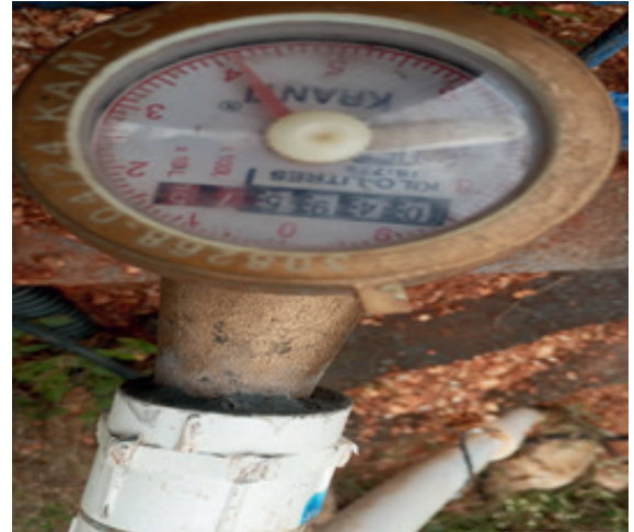
Daily water extraction monitored through flow meter by operations team
